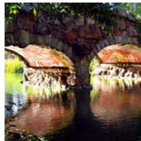
Stone Bridge over Stow L...
