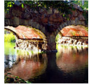
Stone Bridge over Stow L...
